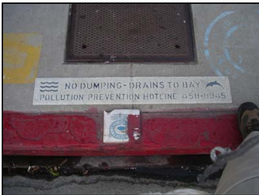
Figure 2. Stenciled storm drain
