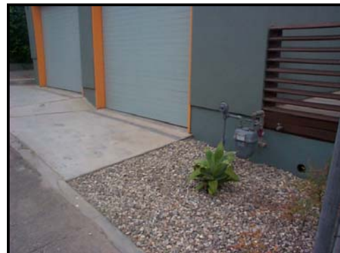
Figure 4. Biofilter for driveway and rooftop
